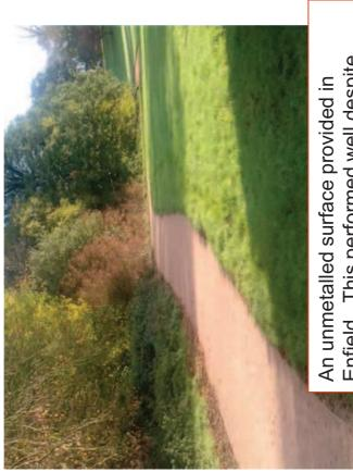
An unmetalled surface provided in Enfield. This performed well despite flooding during extreme weather conditions but areas with a significant gradient and high surface water run-off suffered, which may be an issue for the bridleway.
