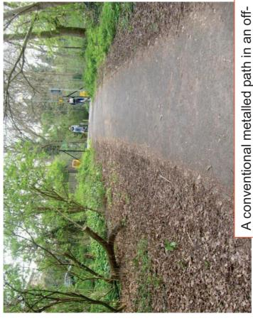
A conventional metalled path in an of road setting. A better surface for cycling but likely to be less preferred for horse-riding.
